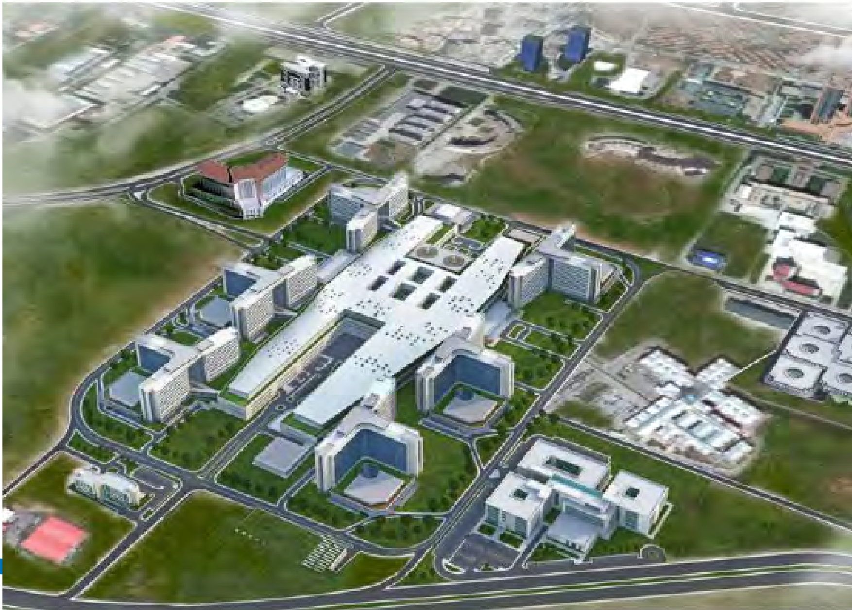
Bilkent Integrated Health Campus Project, Turkey
