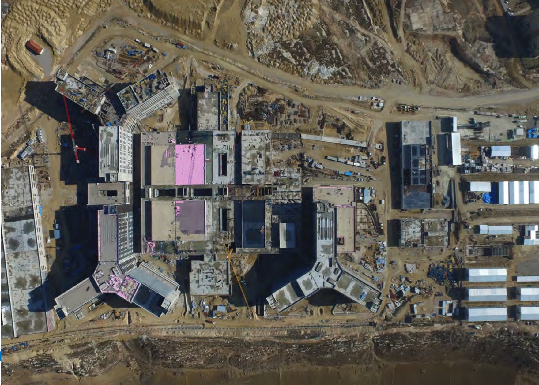
Mersin Integrated Health Campus Project, Turkey
