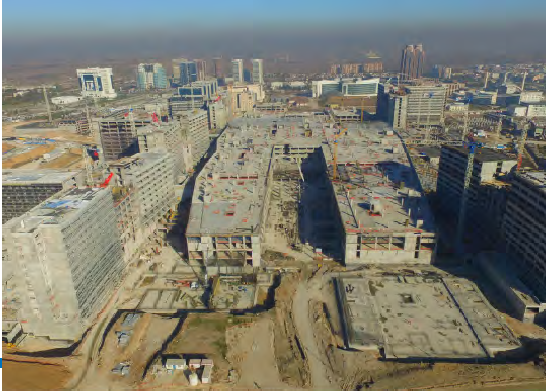
Bilkent Integrated Health Campus Project, Turkey
