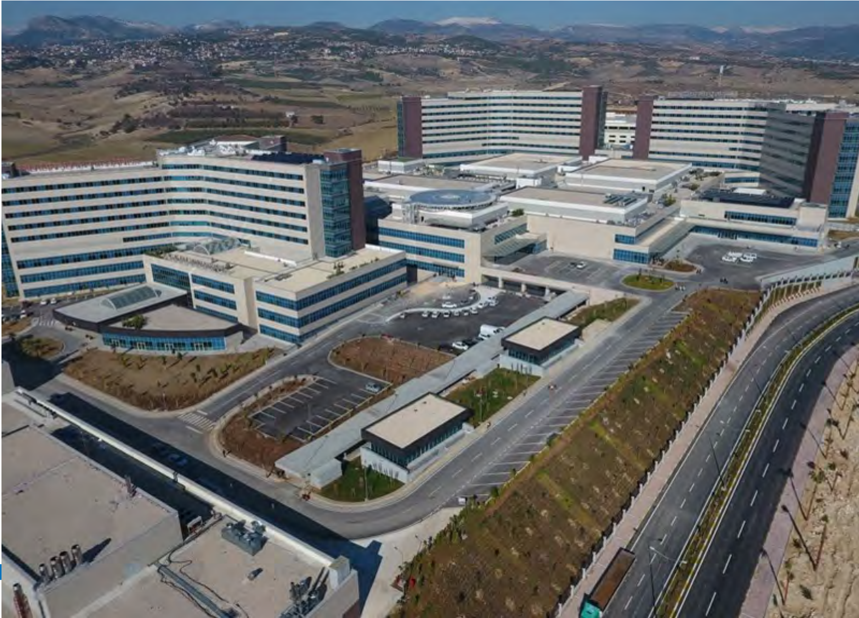
Mersin Integrated Health Campus Project, Turkey
