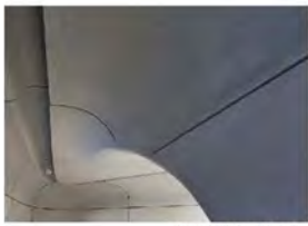
GRC CEILING PANELS
