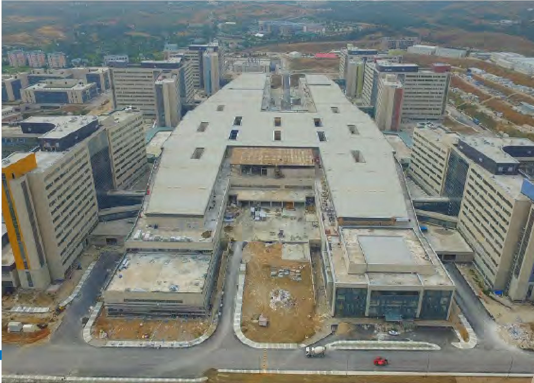
Bilkent Integrated Health Campus Project, Turkey
