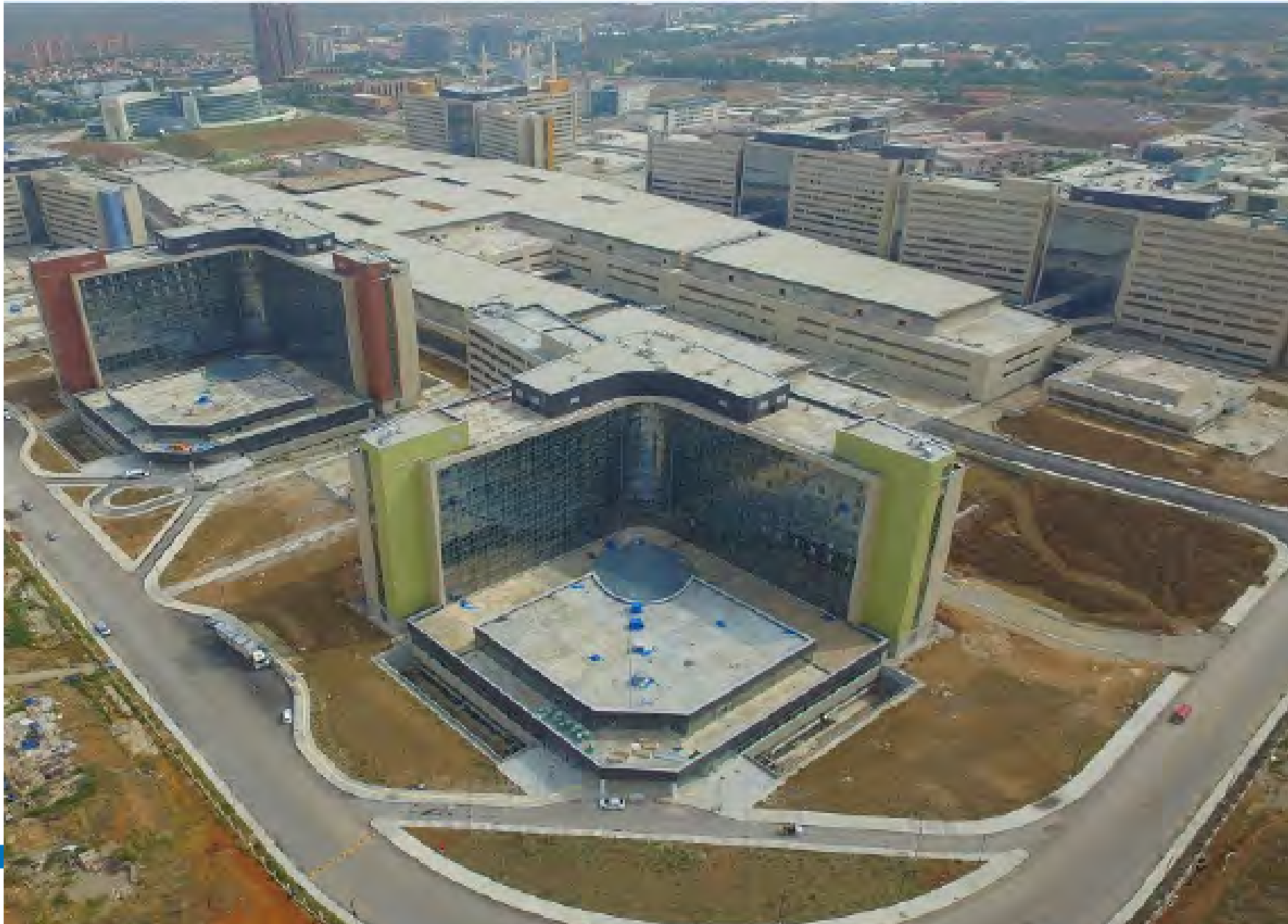
Bilkent Integrated Health Campus Project, Turkey
